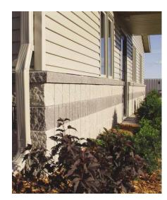
Moderra™ is a revolutionary system for incorporating masonry into building design and construction. Moderra's patented H-channels and brackets allow either vertical or horizontal installation, and require no mortar.
