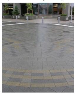
The challenges associated with paver system design and construction in a sub-arctic climate and the demand for very high surface durability due to the winter use of studded tires in Anchorage called for the selection of a system that provides high resistance for horizontal and vertical stresses
