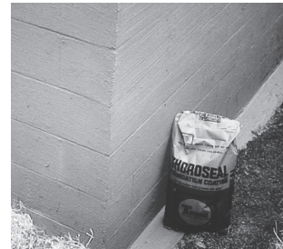
Sealed and waterproofed.
