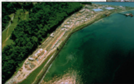
Water and Waste Water Treatment Plants
