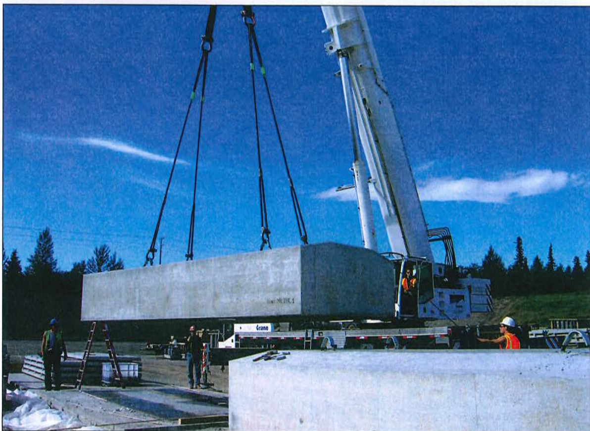
Crane hoists a 30-ton Alaska Railroad bridge component.
