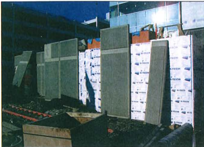
Architectural panels made by Pre-Cast Concrete.
